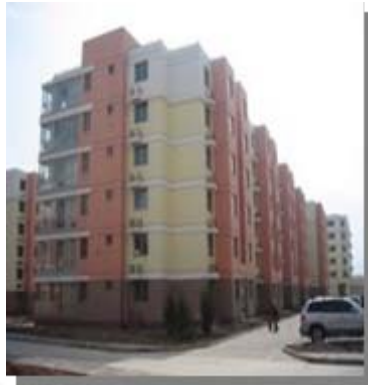
Hohhot Local Revenue, Residence Building
