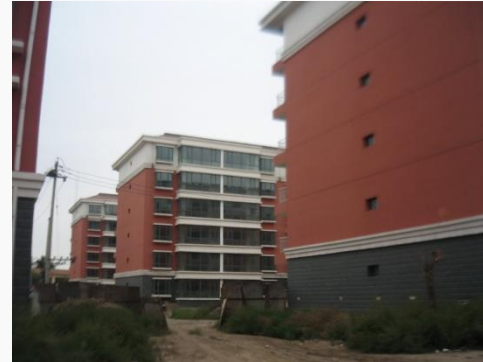
Procuratorate Housing Estates Project Building # 1, #2, #3 On 2010
