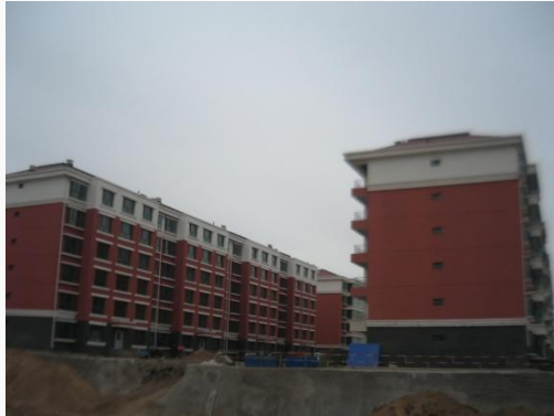
Procuratorate Housing Estates Project Building # 4, #5 On 2010
