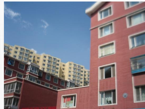
Shuian Renjia Project Eastern Area On 2011
