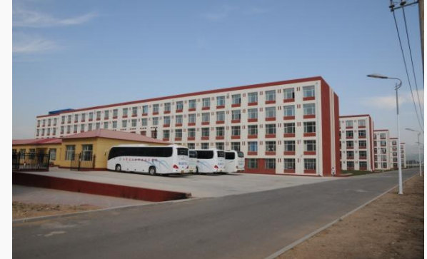
Inner Mongolia Vocational School Buildings On 2008
